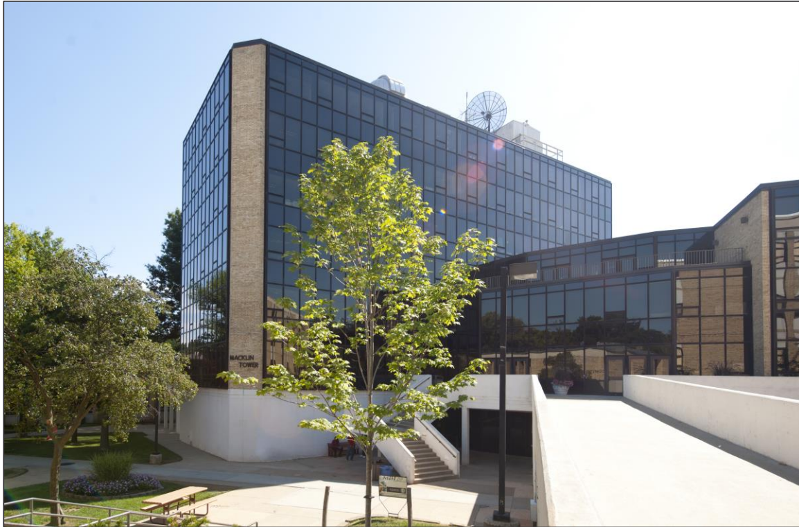
The Gordon and Marilyn Macklin Tower, which houses the library on Montgomery College's Rockville campus. Photo by Pedro "Pete" Vidal.
